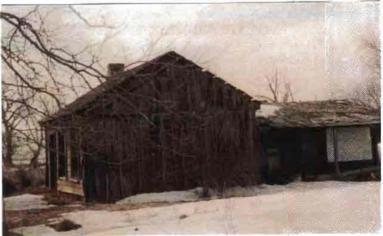
Figure 1. Cabin and addition at back.
