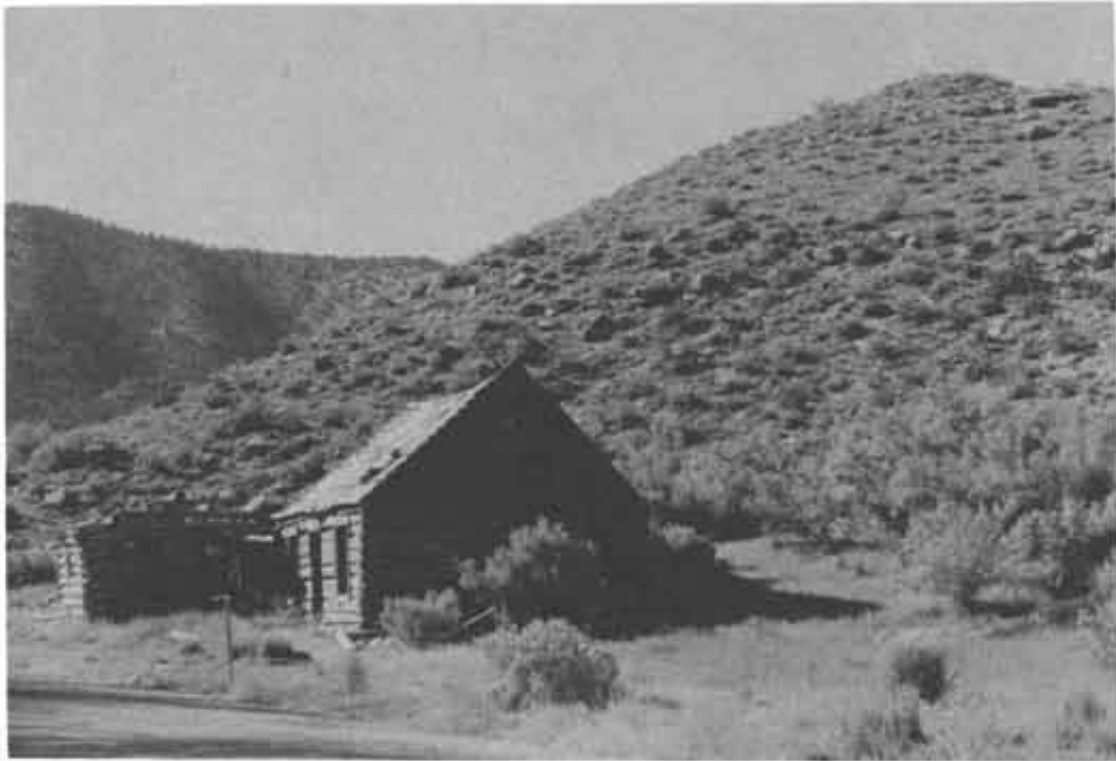
Figure 3. Old post office building at the location currently known as Harper.
